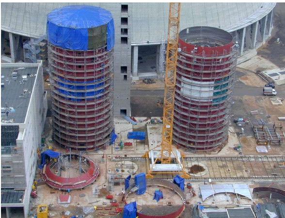
Fabrication of FDG absorber using plates roll-cladded with alloy 59
